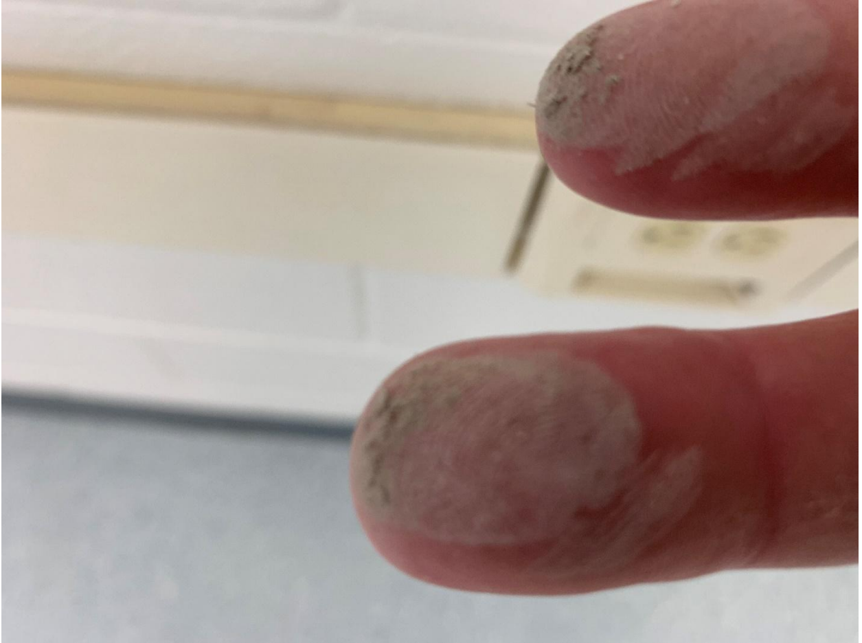
The dirt came from the very visible top of a control box on the wall.
